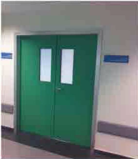
Glass fitted between sandwich sheets
