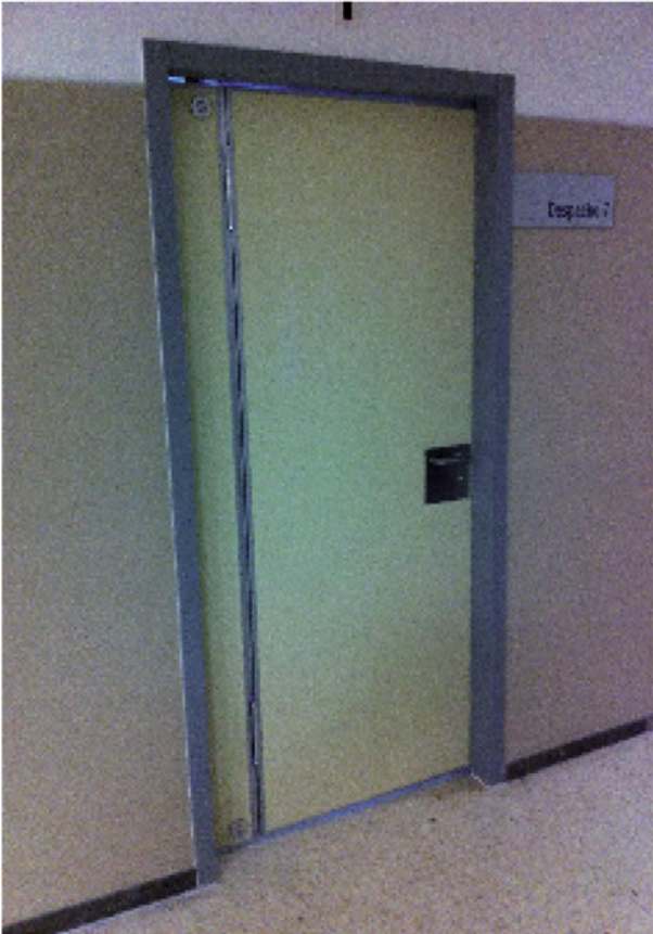
DOOR SEEN FROM OUTSIDE
